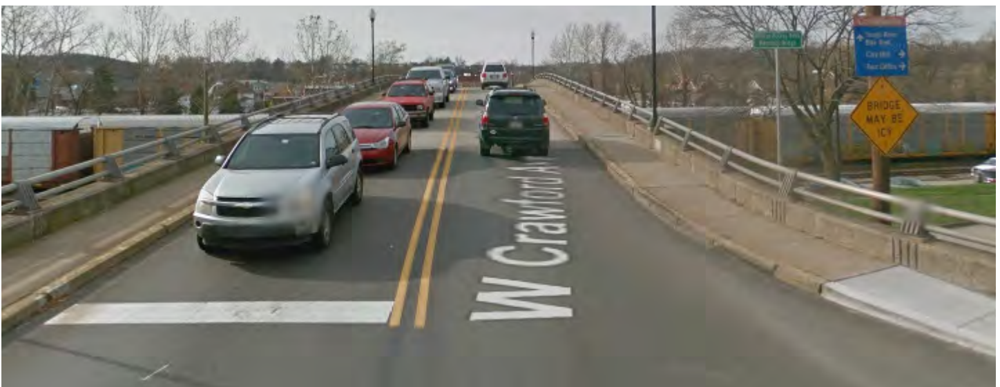
Traffic volume, slope, narrow sidewalks and low safety railing combine for a dangerous Crawford Bridge crossing for pedestrians and cyclists.
